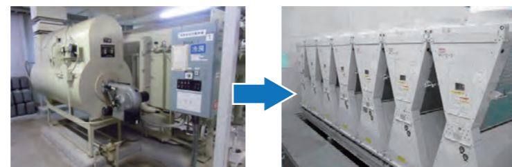
Oil-fired absorption chiller
